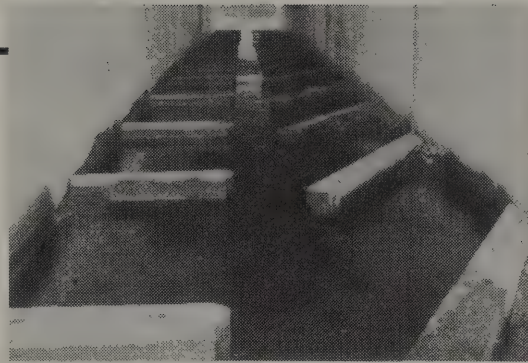
Concrete rectangular culvert with offset baffles bolted to the floor. The baffles were made of treated timber. Without them water velocities would be too high and the depth too shallow during fish migration.
